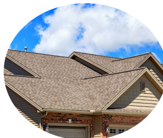
Asphalt Shingle Roof
